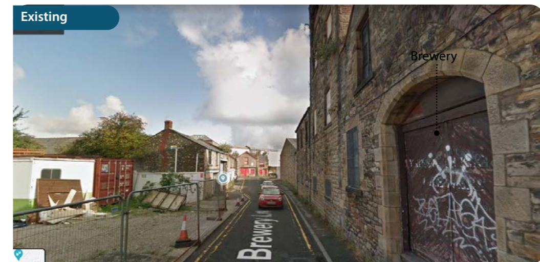
Existing view along Brewery Lane.
