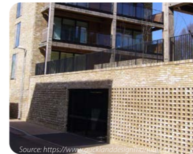
Secure podium parking entrance.
